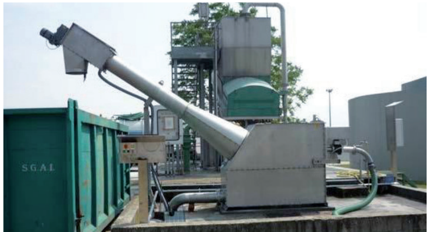
Combined System M2 for tanker imported sludge
