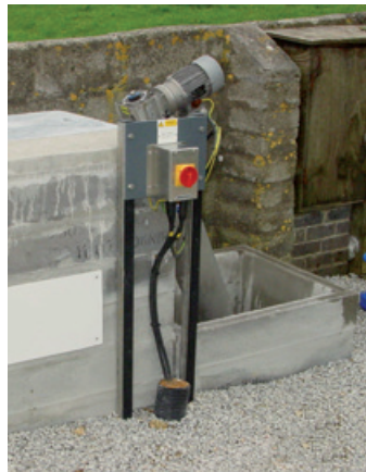
Small wastewater treatment plant
