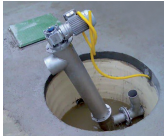
Small village wastewater treatment plant
