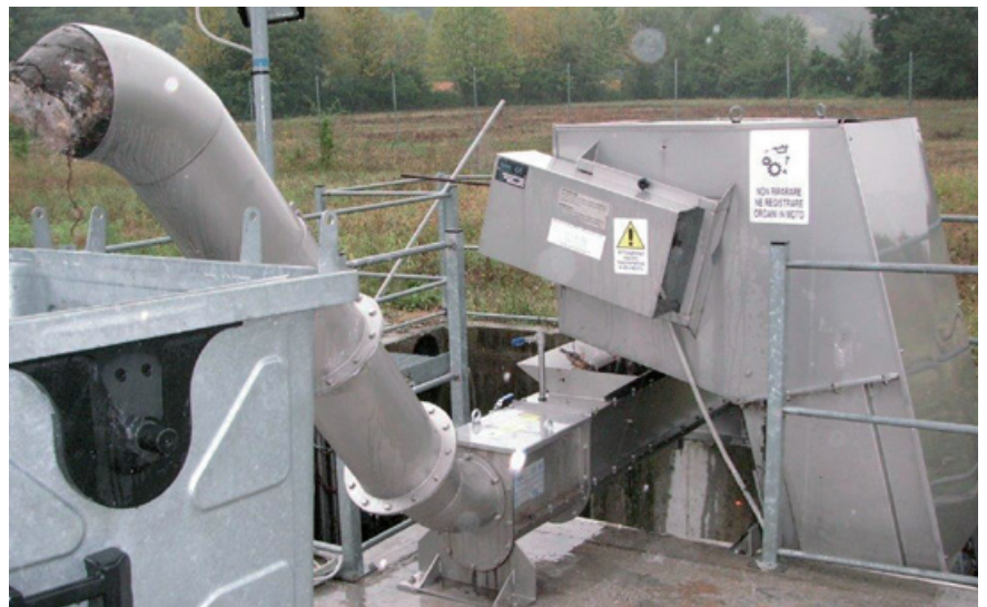
Municipal wastewater treatment plant application
