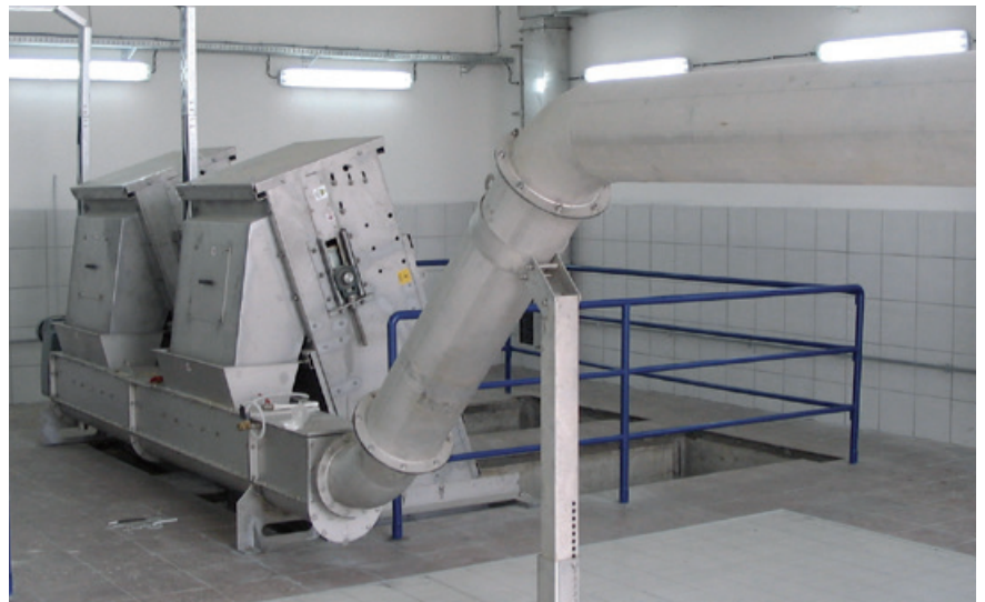
MDX receiving screenings from Bilfinger Johnson Water Technologies MNT Bar Screen
