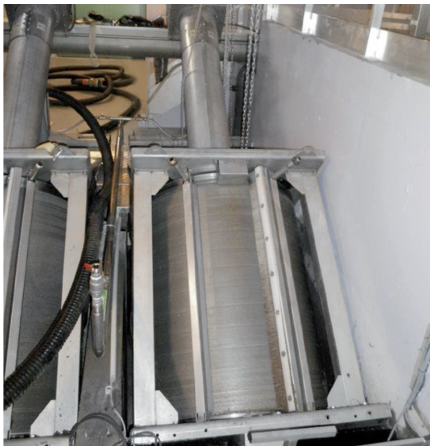
Rotary Drum Screen EMD in channel
